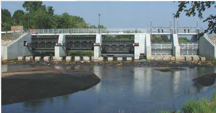
1. Tide gate structure + pumping (tidal + storm)
