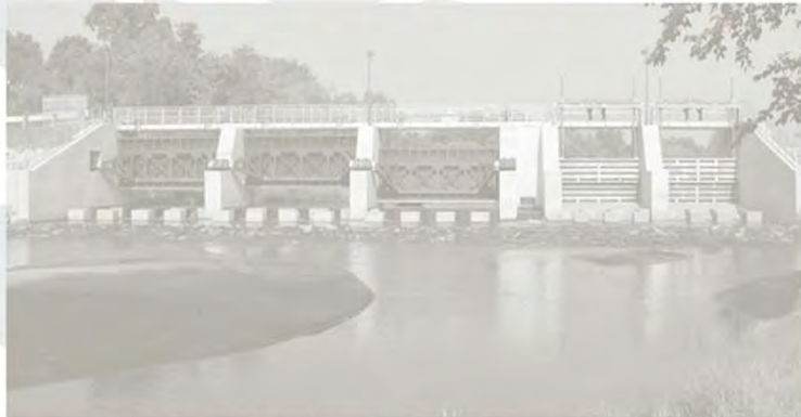
1. Tide-gate structure + pumping (tidal + storm)
